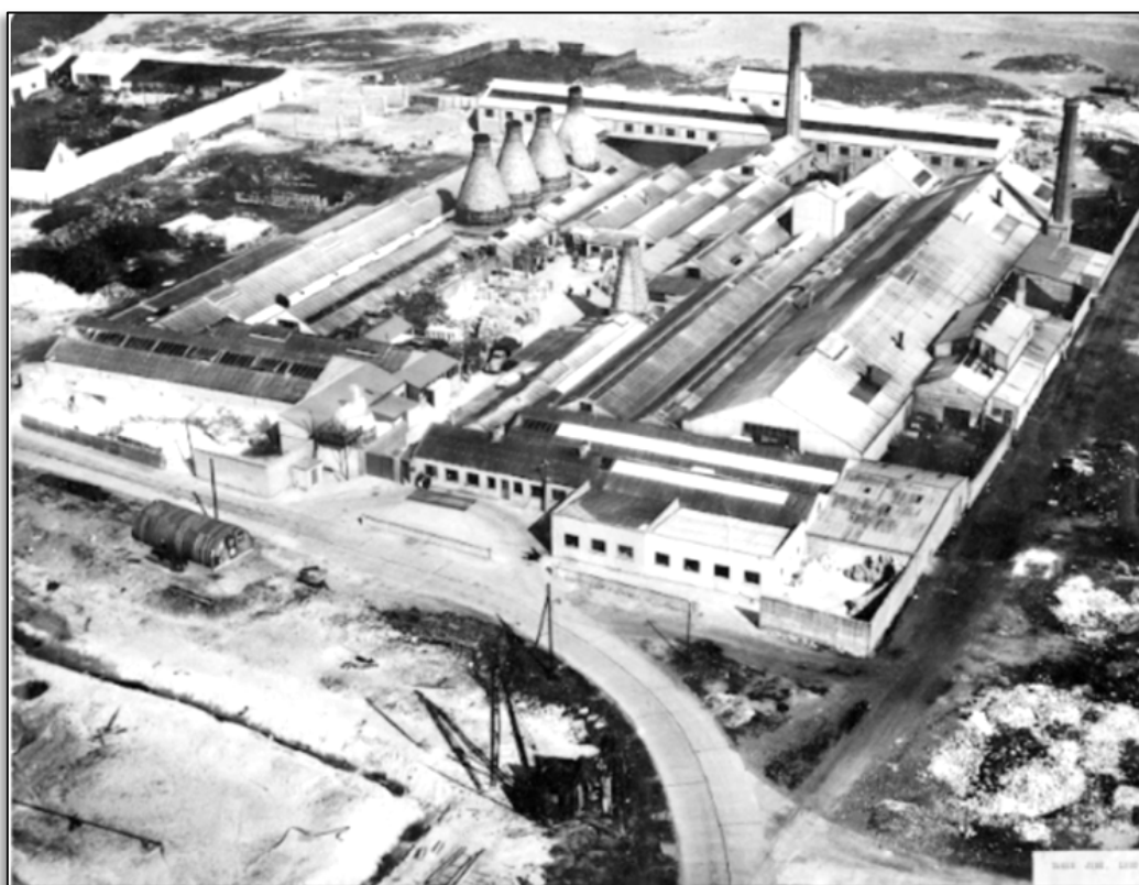
Figure A3.5: Arklow Pottery Factory c. 1950 prior to the demolition of the bottle kilns
